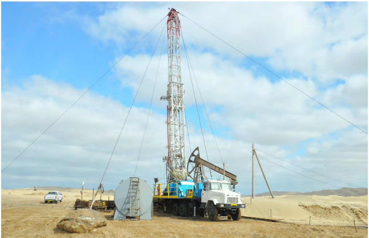
Goturdepe oilfield: Water shut-off jobs by using 80-ton pulling capacity servicing rig
