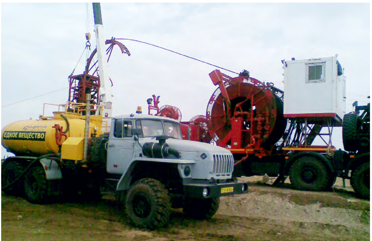
Goturdepe oilfield: CT-conveyed acidizing by employing acid-proof pumper
