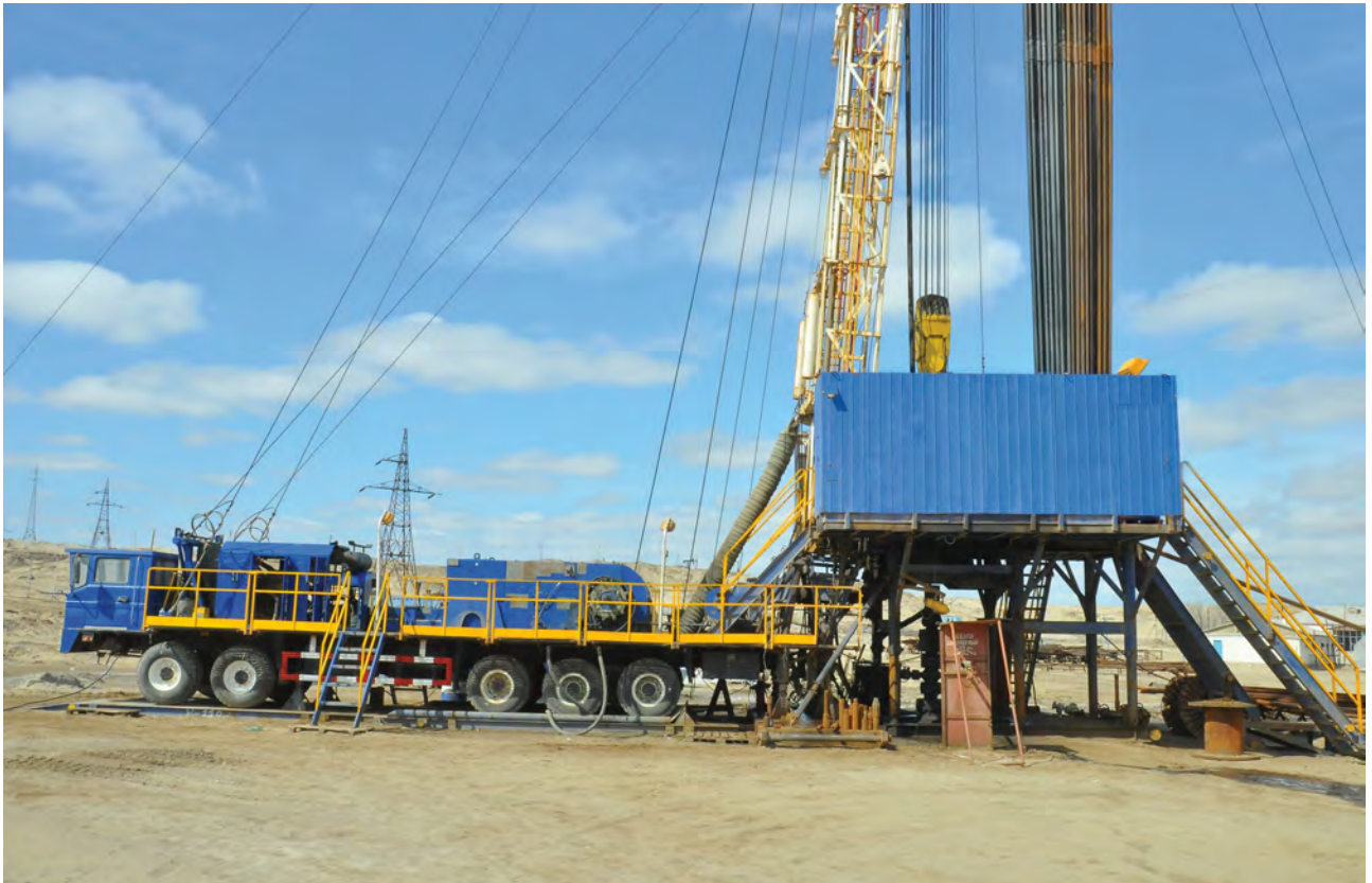
Goturdepe oilfield: Well workover in abnormal operating conditions by using a workover rig (125 ton load capacity)
